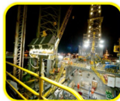
Petrol Process Factory
